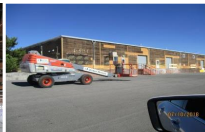
SIAD Siding Replacement
