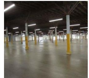
SIAD Structural REPAIR
