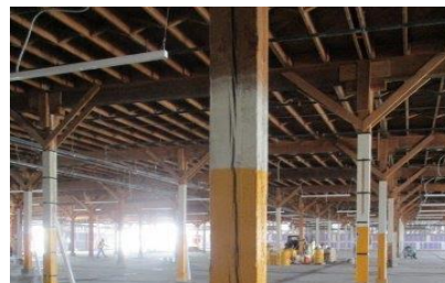
SIAD Structural REPAIR
