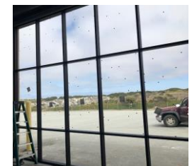
USAR Warehouse REMODEL
