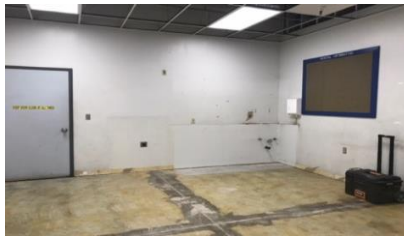
DDJC Breakroom RENOVATION
