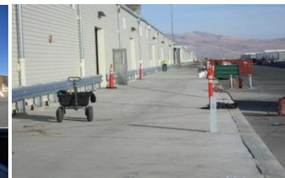
SIAD Siding Replacement
